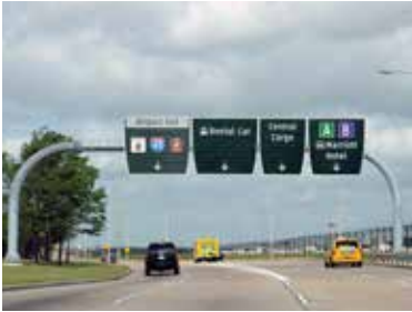
Houston, TX - Airport TXDOT Roadway Signage
